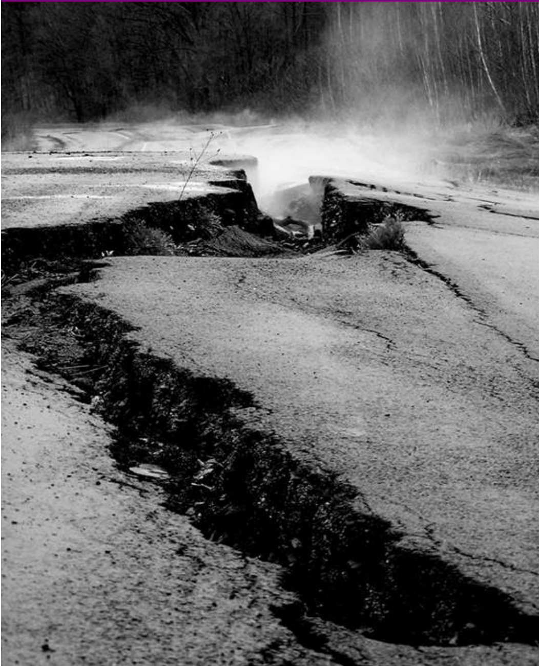
Figure 20.1 This underground mine fire in Centralia, Pennsylvania, could burn for over a century. (Photo courtesy of jesiehart/flickr)
